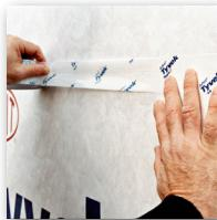
**DuPont™ Tyvek® Tape, DuPont™ Tyvek® Wrap Caps and DuPont™ Residential Sealant, integral parts of DuPont™ Tyvek® Weatherization Systems.**
