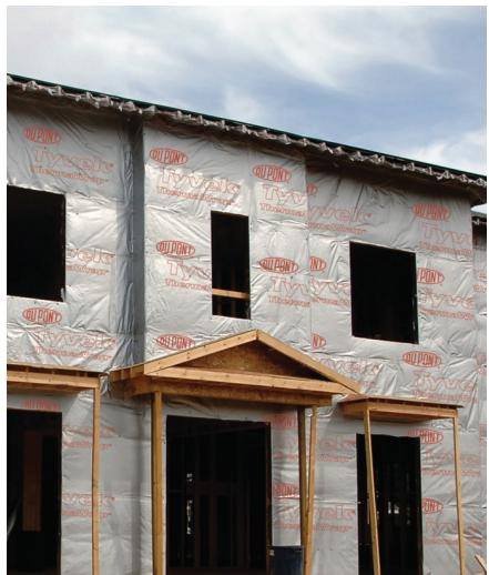
DuPont™ Tyvek® ThermaWrap™ is a high-performance barrier that helps increase the thermal performance of a wall system by managing radiant heat flow.
