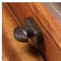
turn knob lock on the bottom rail of the bottom sash in the closed position
